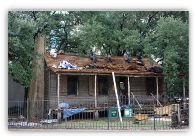
Internal gutters on the *1868 Pillot House* were repaired in October 2016. Paul Gollub Roofing cleaned and soldered the gutters to eliminate leaking and repaired and replaced rotten wood at the soffits on the front of the building. In April 2017, the 1891 St. John Church received a complete exterior cleaning along with touch-up painting on the interior. Earlier in the year, the original front doors were repainted as well.
